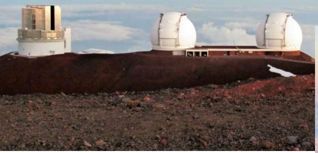
Both Keck telescopes feature 10 meter primary mirrors. The combination of an excellent site, large optics and innovative instruments has created the two most scientifically productive telescopes on Earth.
